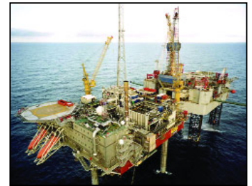
In the case of two accommodation modules for platforms in the Gulf of Mexico, an EPC found that CADPIPE could meet the challenge of multiple disciplines.
